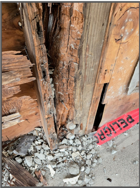
Photos of dry rot near the elevator shaft at 3711 Terra Granada, Entry 6. Another example of the structural damage uncovered in the building rehabilitation project.
