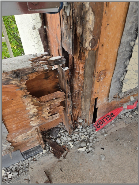
Photos of dry rot near the elevator shaft at 3711 Terra Granada, Entry 6. Another example of the structural damage uncovered in the building rehabilitation project.
